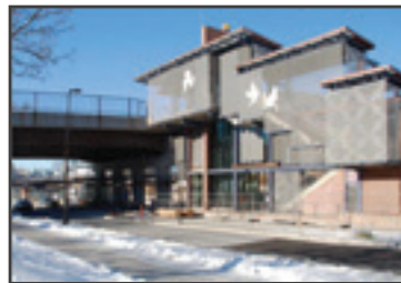
West Bank Station between 19th and Cedar.
